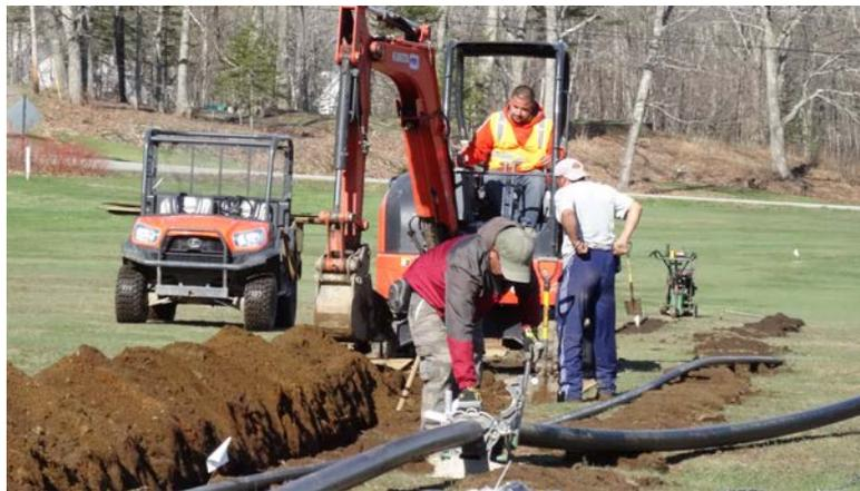
**Photo 2 – Detail of Splicing the Water Pipe**
