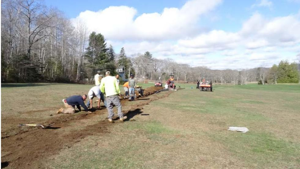
**Photo 1 – Installation of Water Lines on Fairway 5**
